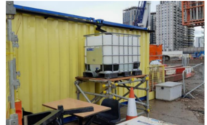
Rainwater harvesting on a UK construction site
